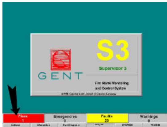
Figure 31-2 Display after fire is acknowledged jnpic2
